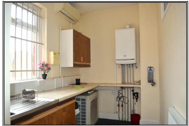
First Floor Kitchen
